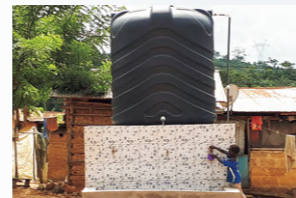
Constructed well with a cistern
