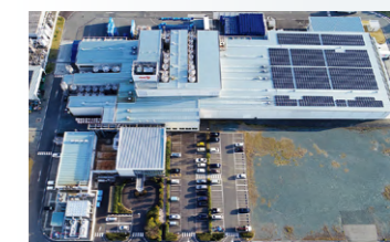
Solar power generation equipment at Tokai Meiji Co., Ltd.
