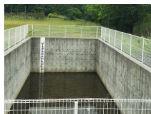
Rainwater storage facility
