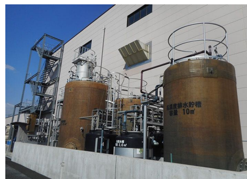
Methane fermentation process
