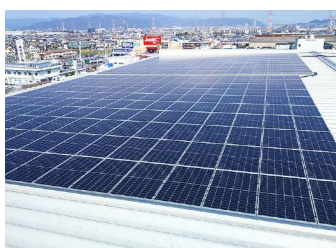
Meiji Oils and Fats (April 2020 Operation)
