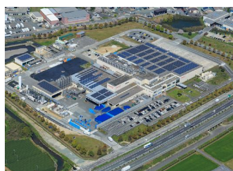
Kyushu Plant (April 2020 operation)
