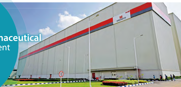
Unit 7, a new plant for Medreich Limited
