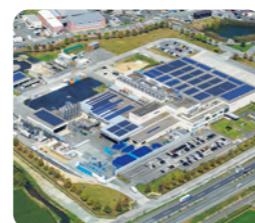
Solar power generation equipment, which started operation in April 2020 at Meiji's Kyushu Plant
