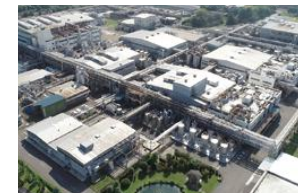
Panoramic view of Gifu Plant
