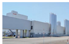
Exterior of the New Hokkaido Plant
