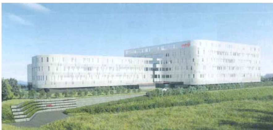
Image of Completed New Research Facility
