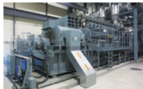
Co-generation system at Tokachi Plant of Meiji Co., Ltd.
