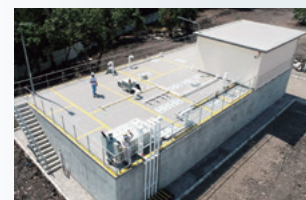
PT. Meiji Indonesian Pharmaceutical Industries' activated sludge treatment system
