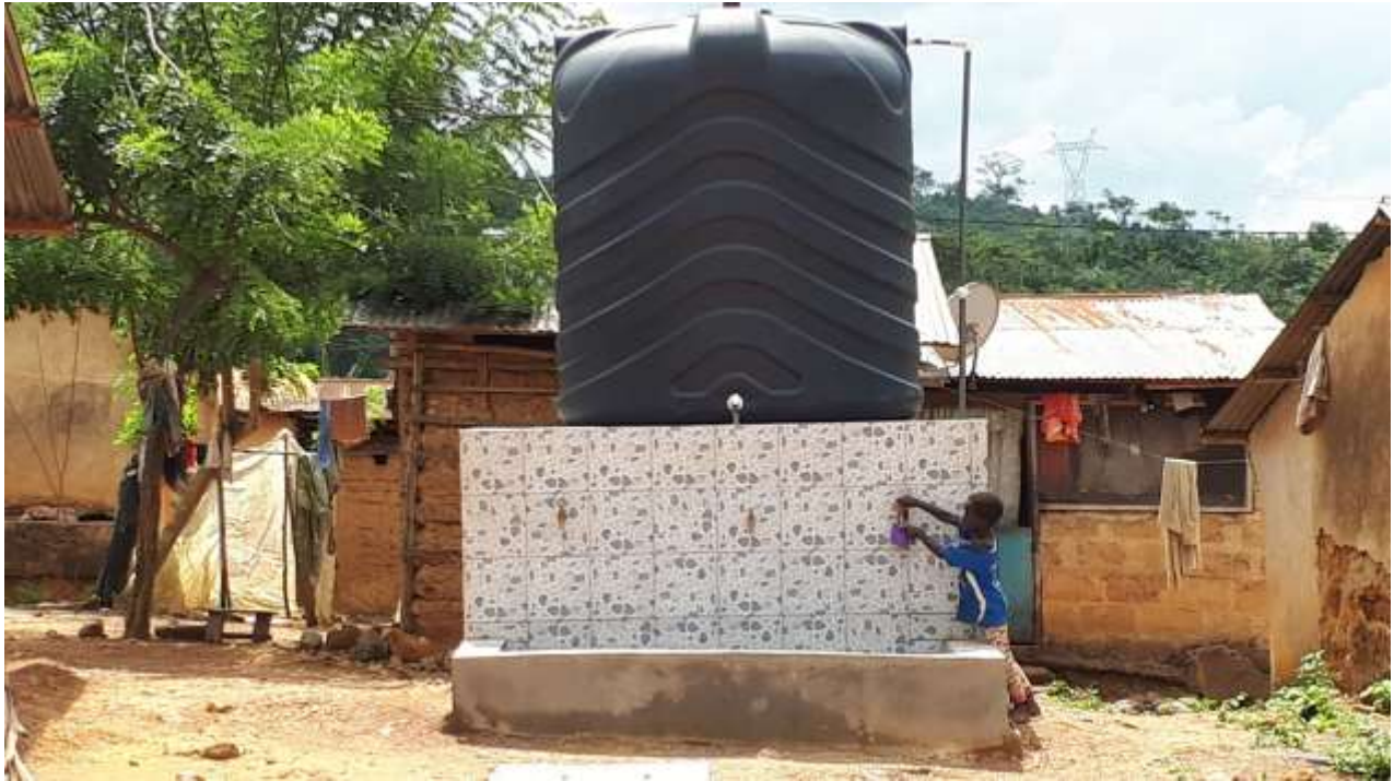
New Borehole in Ayensukrom Society
