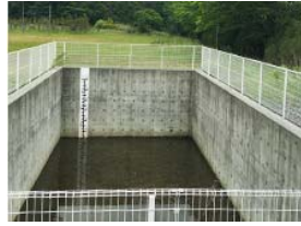
Rainwater storage facility
