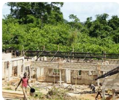
Construction of an elementary school
