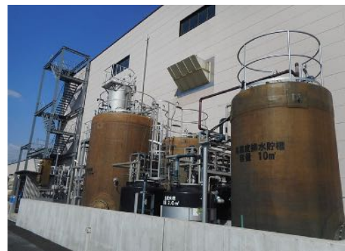
Methane fermentation process
