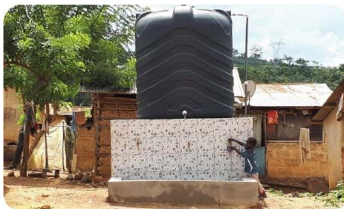
Built a well with a water storage tank
