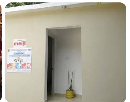
Newly established toilets
