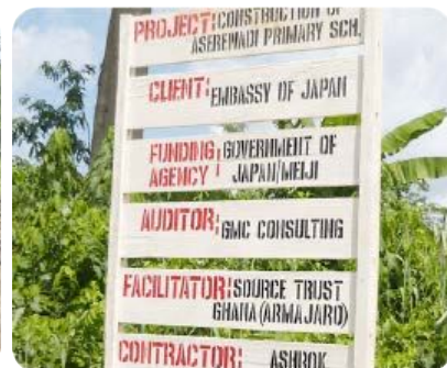
Signage of the elementary school construction project
