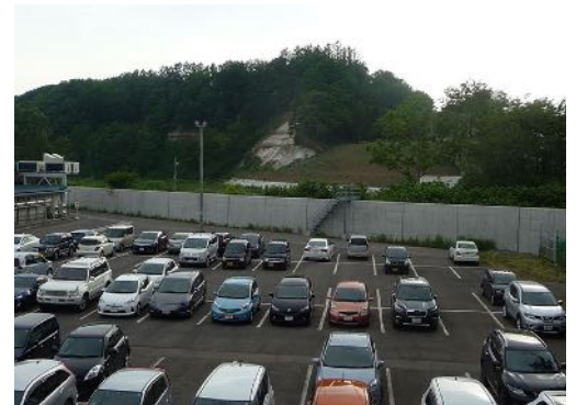
Nihon Kanzume water barrier
