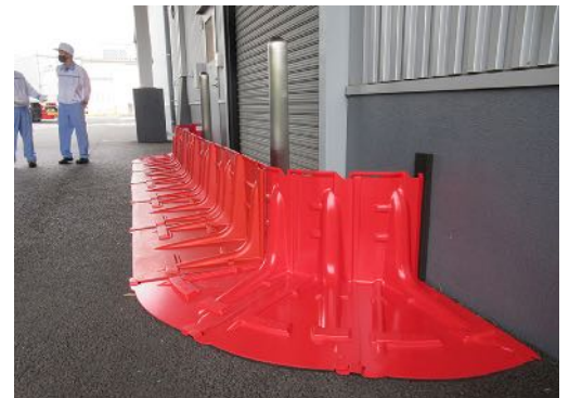
Provisional water stops in Meiji Seika Pharmatech Co., Ltd.
