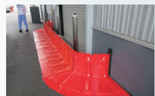
A drill to set up provisional water stops held at Meiji Seika Pharma Co., Ltd.'s Odawara Plant
